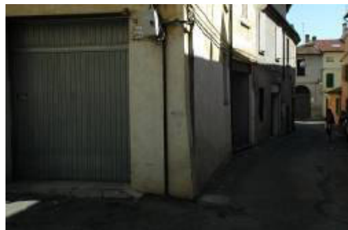
Fig. 17 – Muro a scarpa in via Costa
